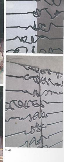
8-13. Kleine Rittergasse 11: Prototypes and trial assembly of the façade.
